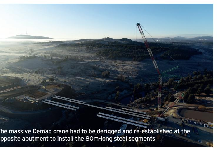
The massive Demag crane had to be derigged and re-established at the opposite abutment to install the 80m-long steel segments
