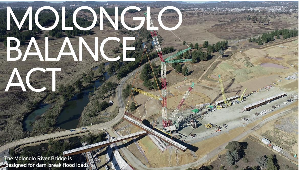
The longest weathering steel span in the southern hemisphere is now in place across Canberra's largest river. **Irene Scott** explains why the bridge girder was fully redesigned and how the crossing's massive steel sections were installed
